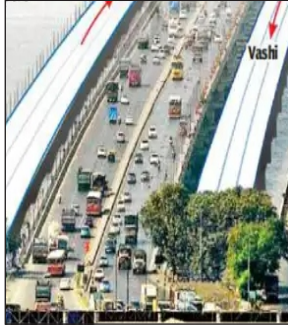
VASHI CREEK BRIDGE
