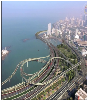
L & T COASTAL ROAD PROJECT
